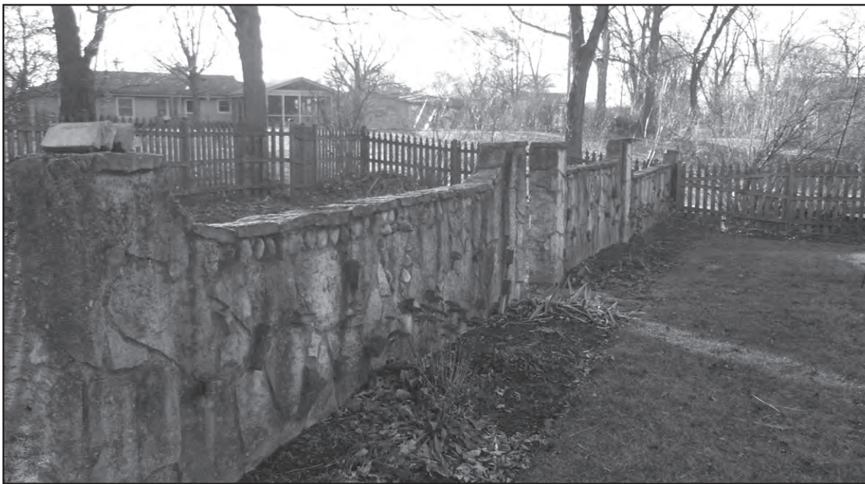
the flagstone wall from the original Model electric Home of 1929 can still be seen at 323 West Crystal lake avenue in Crystal lake
