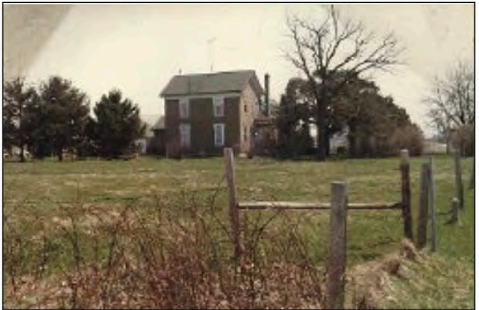
Not much was left of an 1850s two-story farm house that burned down in January. Dr. David Hucek and his wife will rebuild a two-story 21st Century house on a new foundation.
